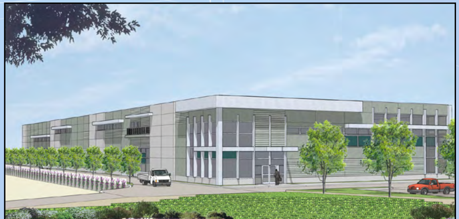
Desalination project in Carlsbad.
